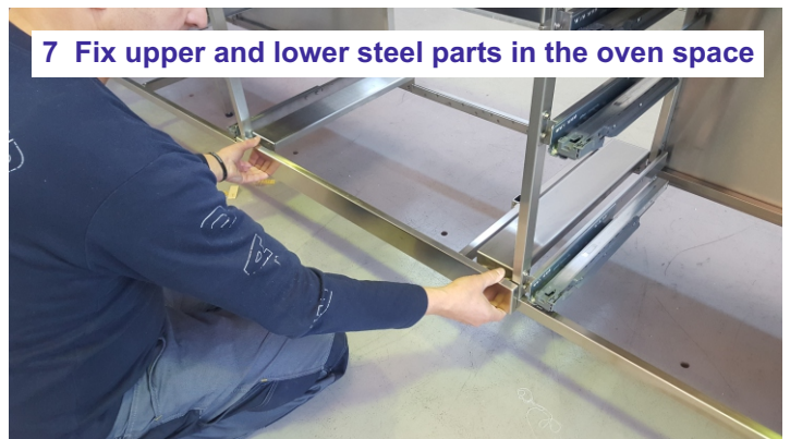
7 Fix upper and lower steel parts in the oven space
