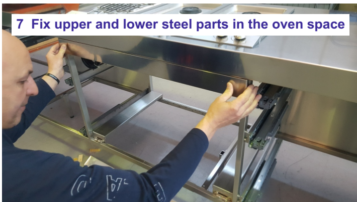
7 Fix upper and lower steel parts in the oven space
